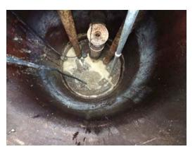
Same wet well just 10 minutes following the start-up of the *WET WELL*WIZARD. Note that the float switch has already repositioned itself.
