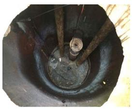
A 5' diameter wet well with a 2.5 foot thick FOG cap. Note the float switch lying on top – causing pump short-cycling
