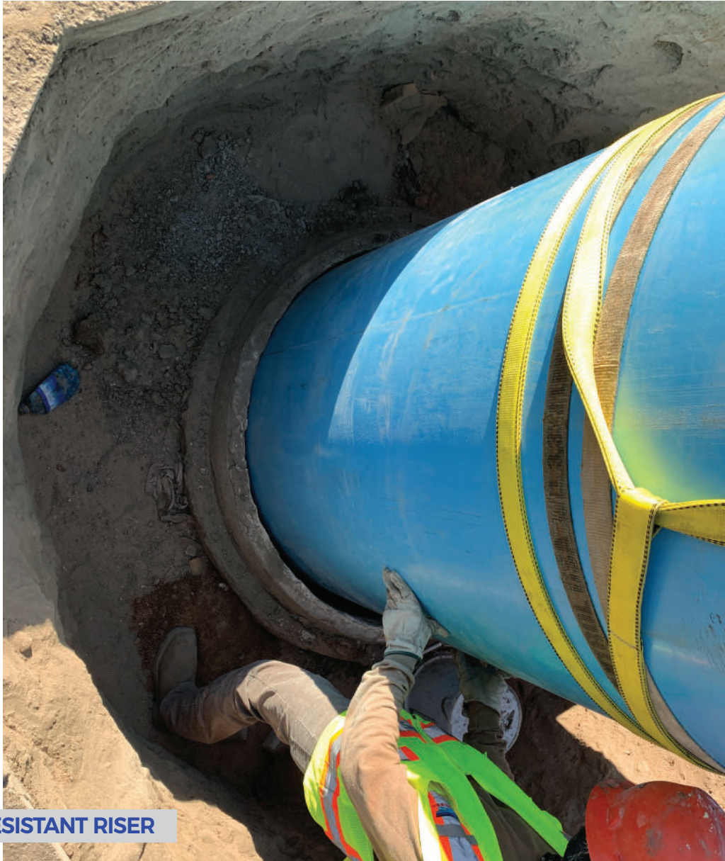
LOWER AWWA C900 RISER ONTO BASE
