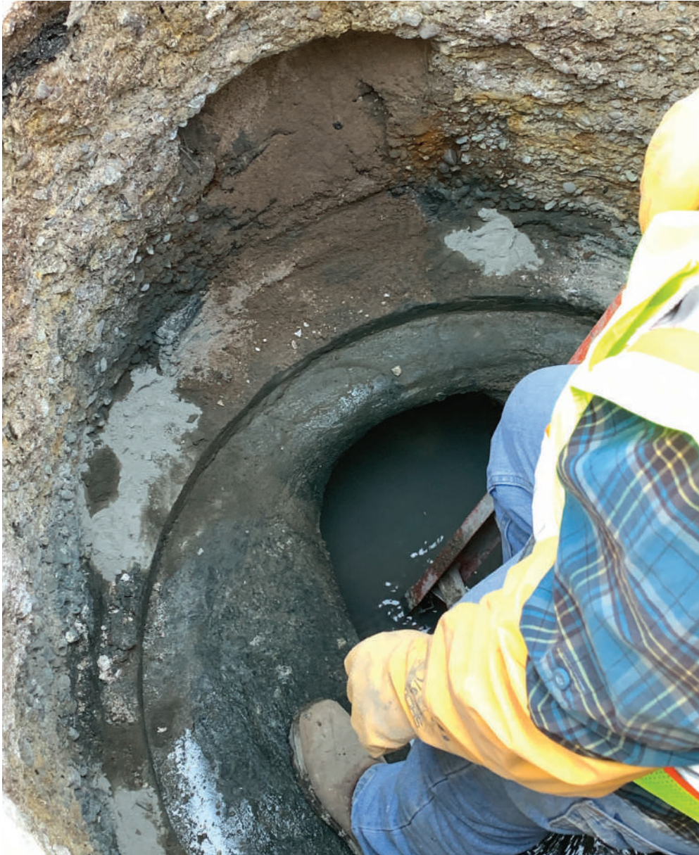
REBUILT BENCH
