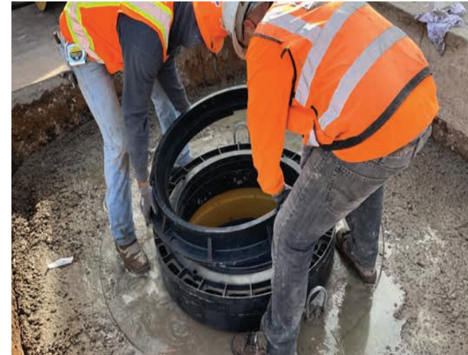
INSTALLATION WITH HDPE GRADE RINGS
