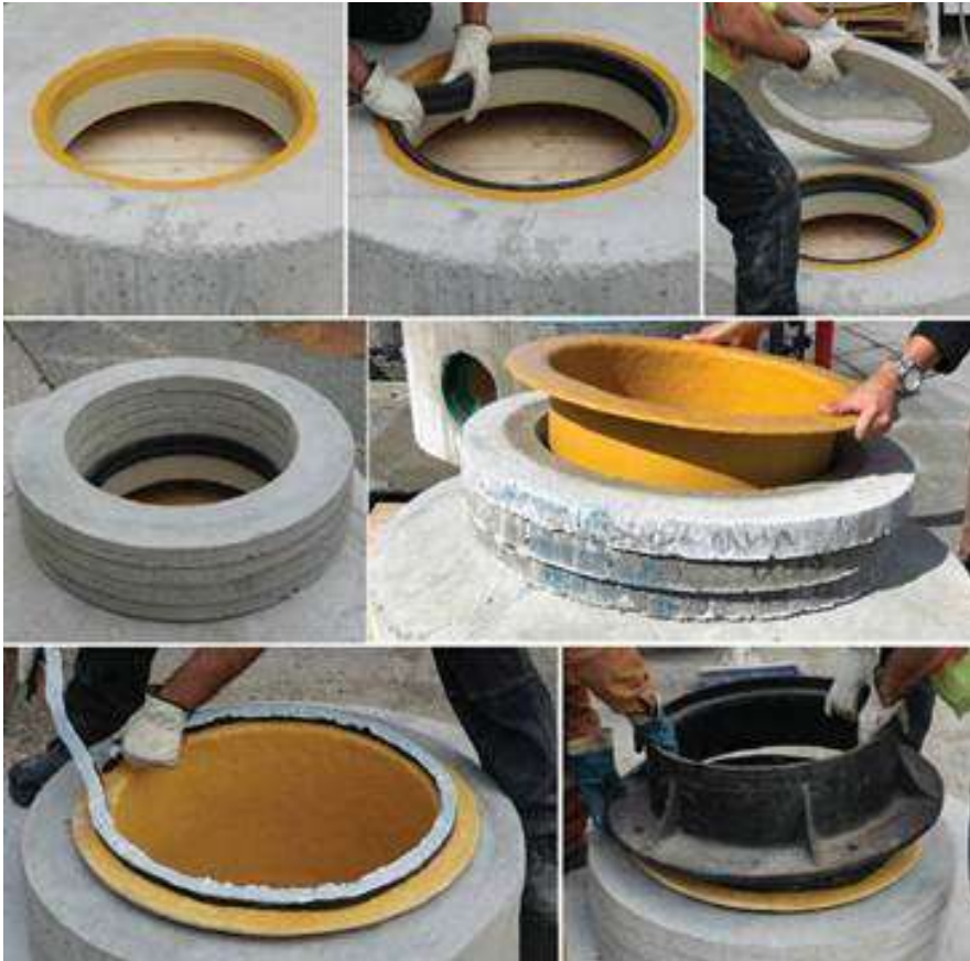
INSTALLATION WITH CONCRETE GRADE RINGS
