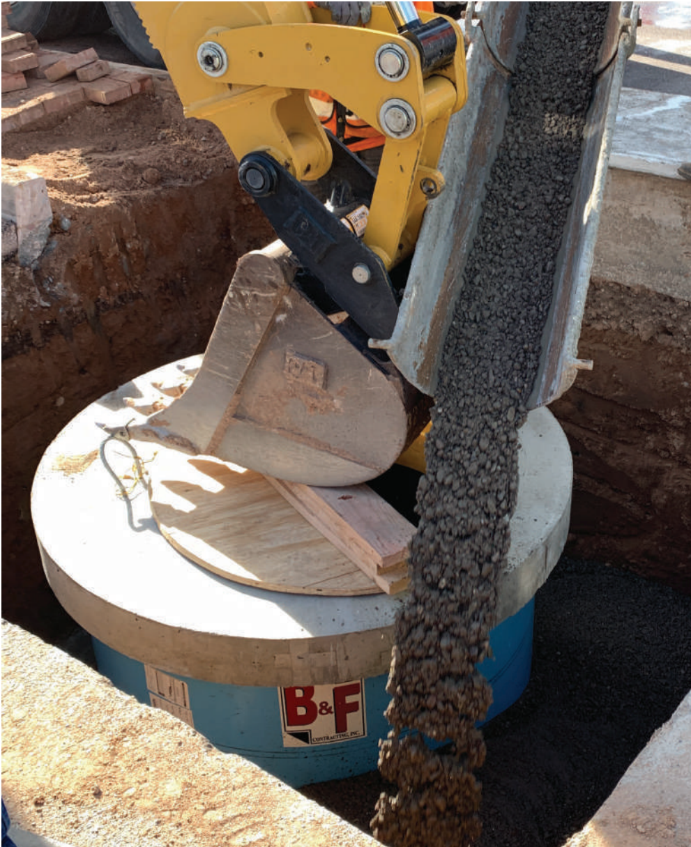
BACKFILL
