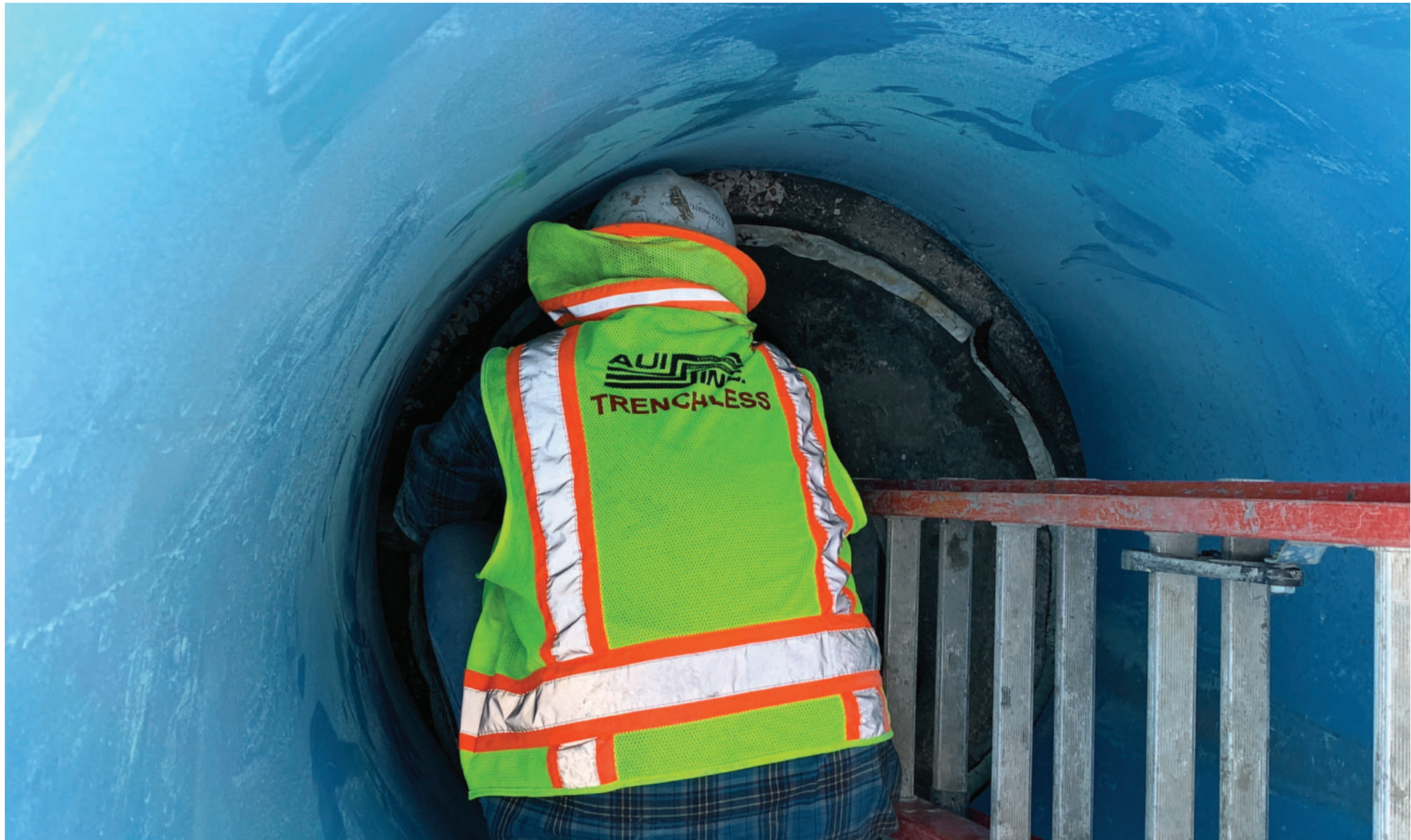
SETTING THE MASTIC ON THE BENCH TO RECEIVE THE PVC RISER
