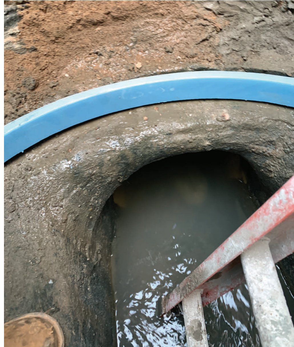
ASSURING THE RISER FIT THE REBUILT BENCH
