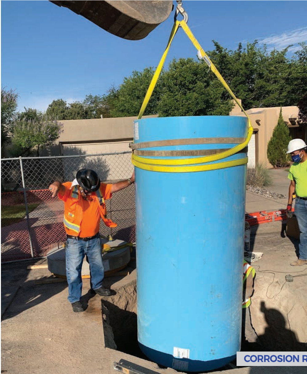
LOWER AWWA C900 RISER ONTO BASE
