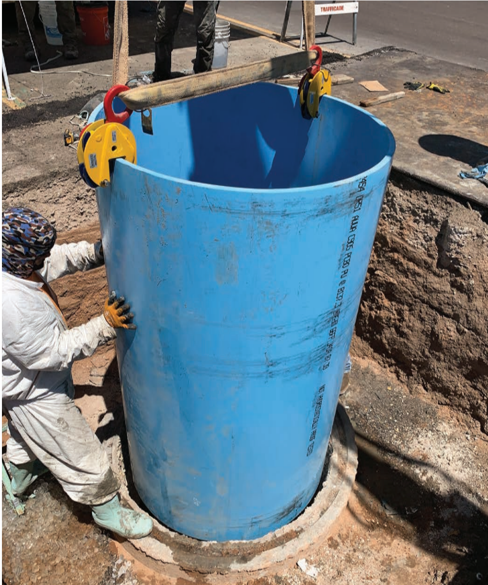
LOWER PVC RISER INTO MH
