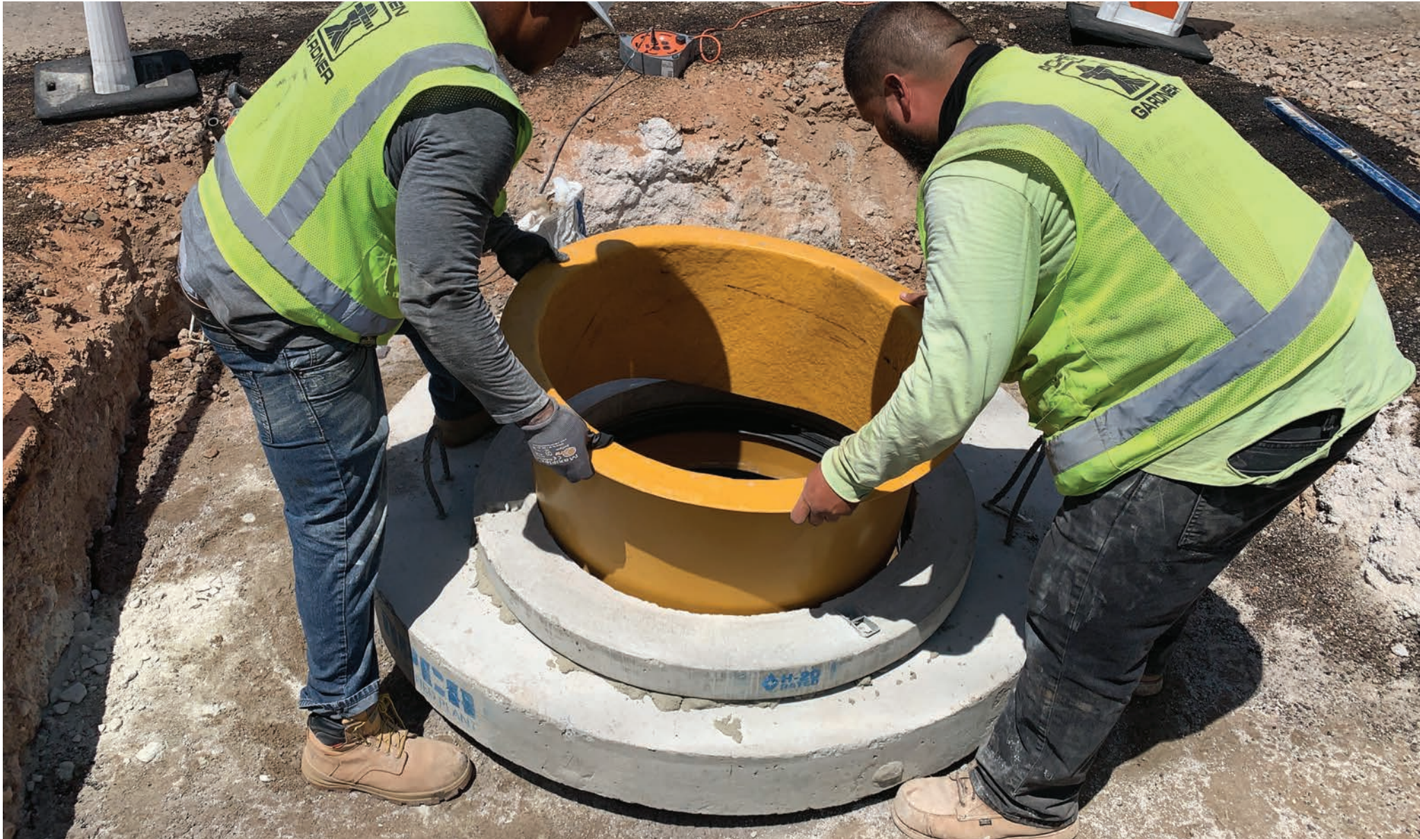
INSERT TELESCOPIC ACCESS COLLAR TUBE
