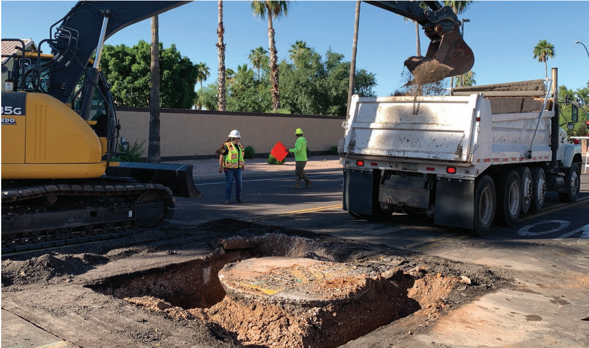
EXCAVATE AND REMOVE EXISTING FLAT TOP OR CONE TOP
