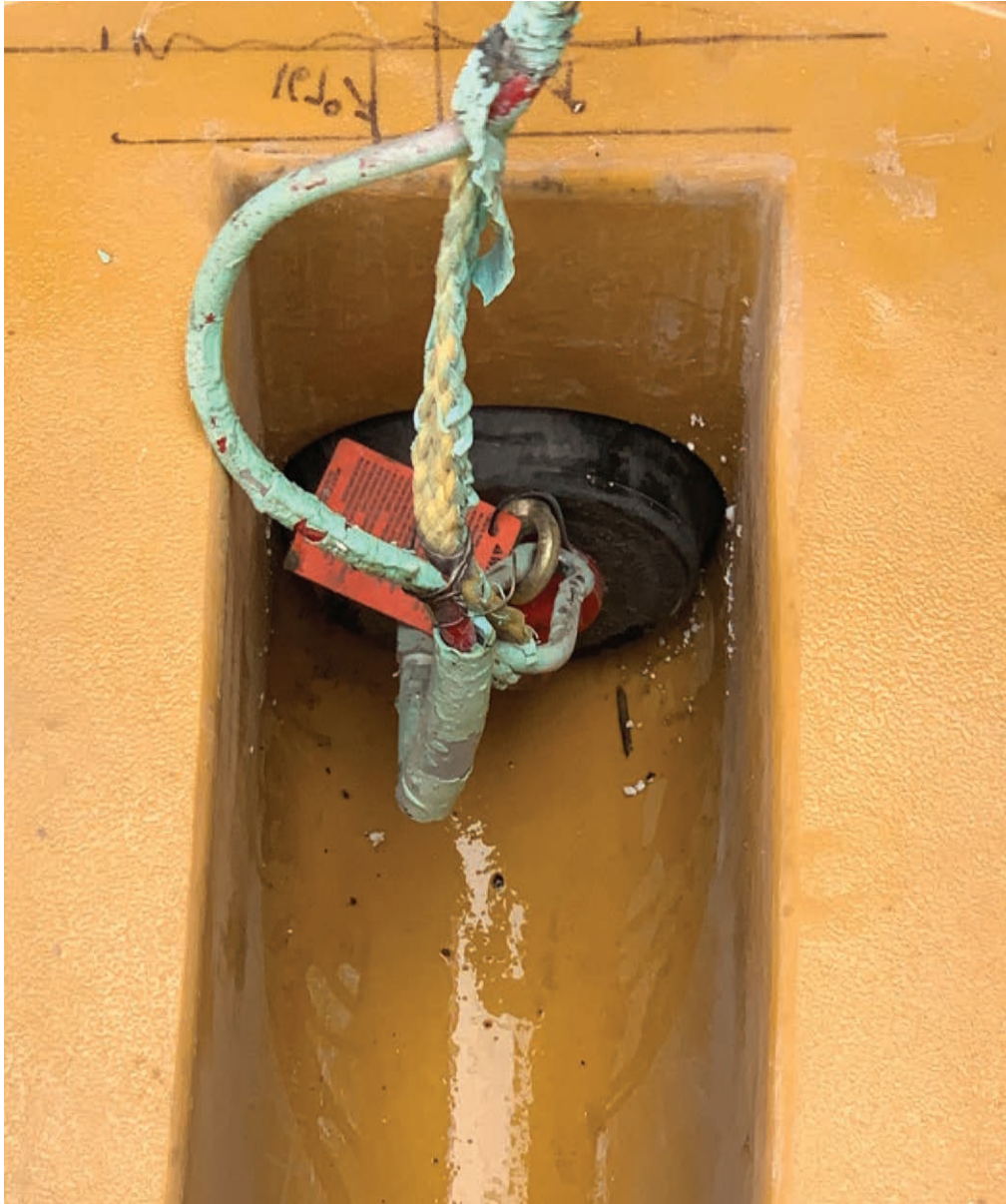
PIPE PENETRATION TO BE SEALED WITH INFLATABLE PLUGS
