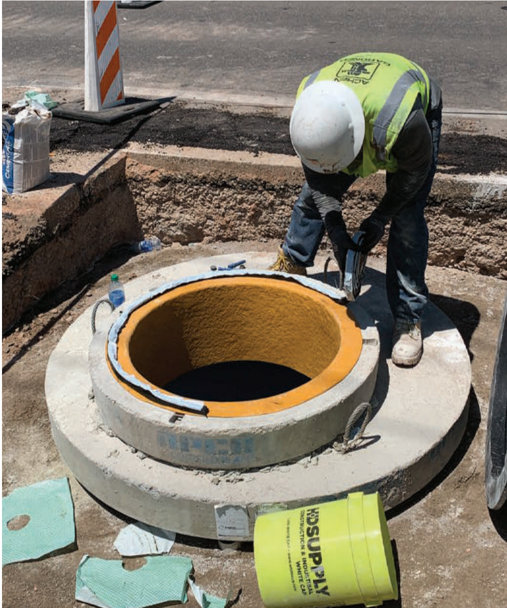
PLACE BUTYL RUBBER SEALANT ON TOP FLANGE OF TAC
