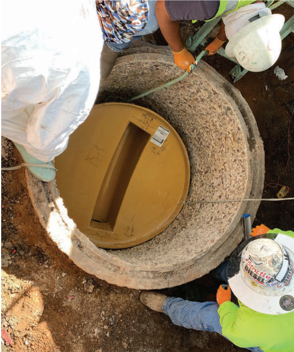
LOWER BASELINER INSERT INTO MANHOLE
