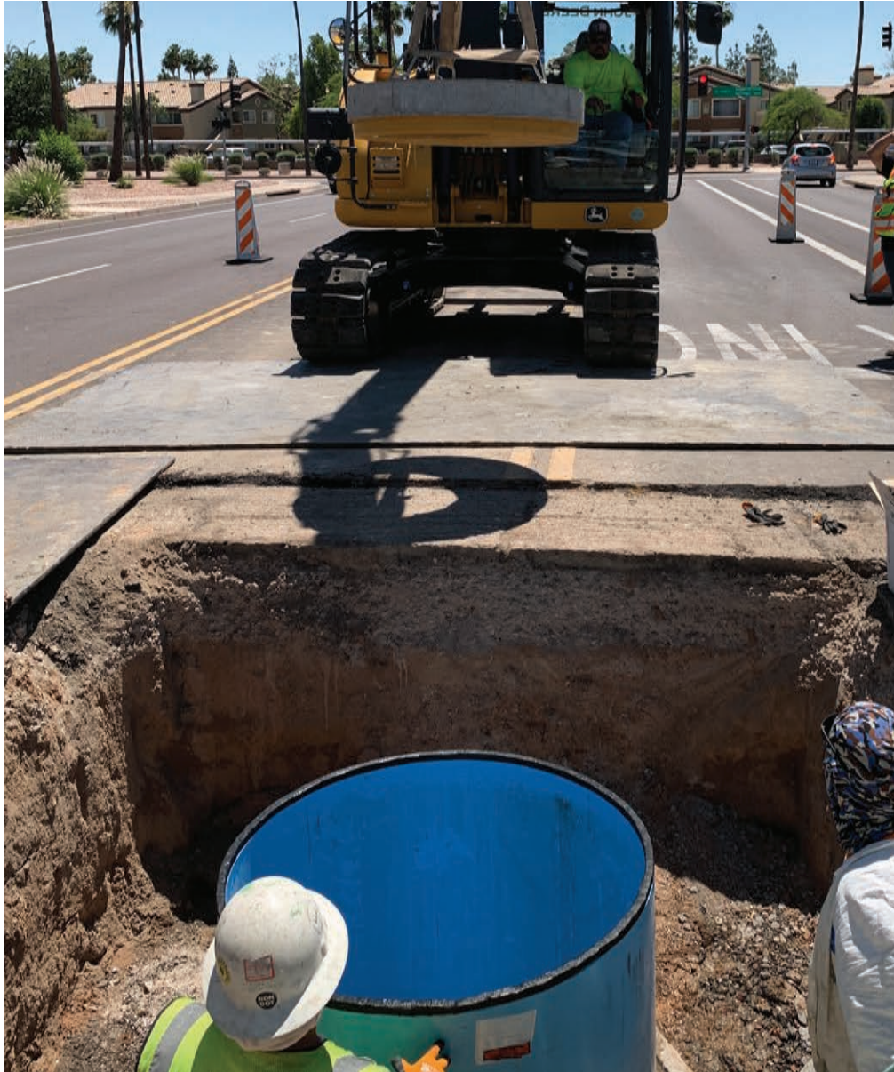
LOWER FRP LINED PRECAST LID ONTO RISER
