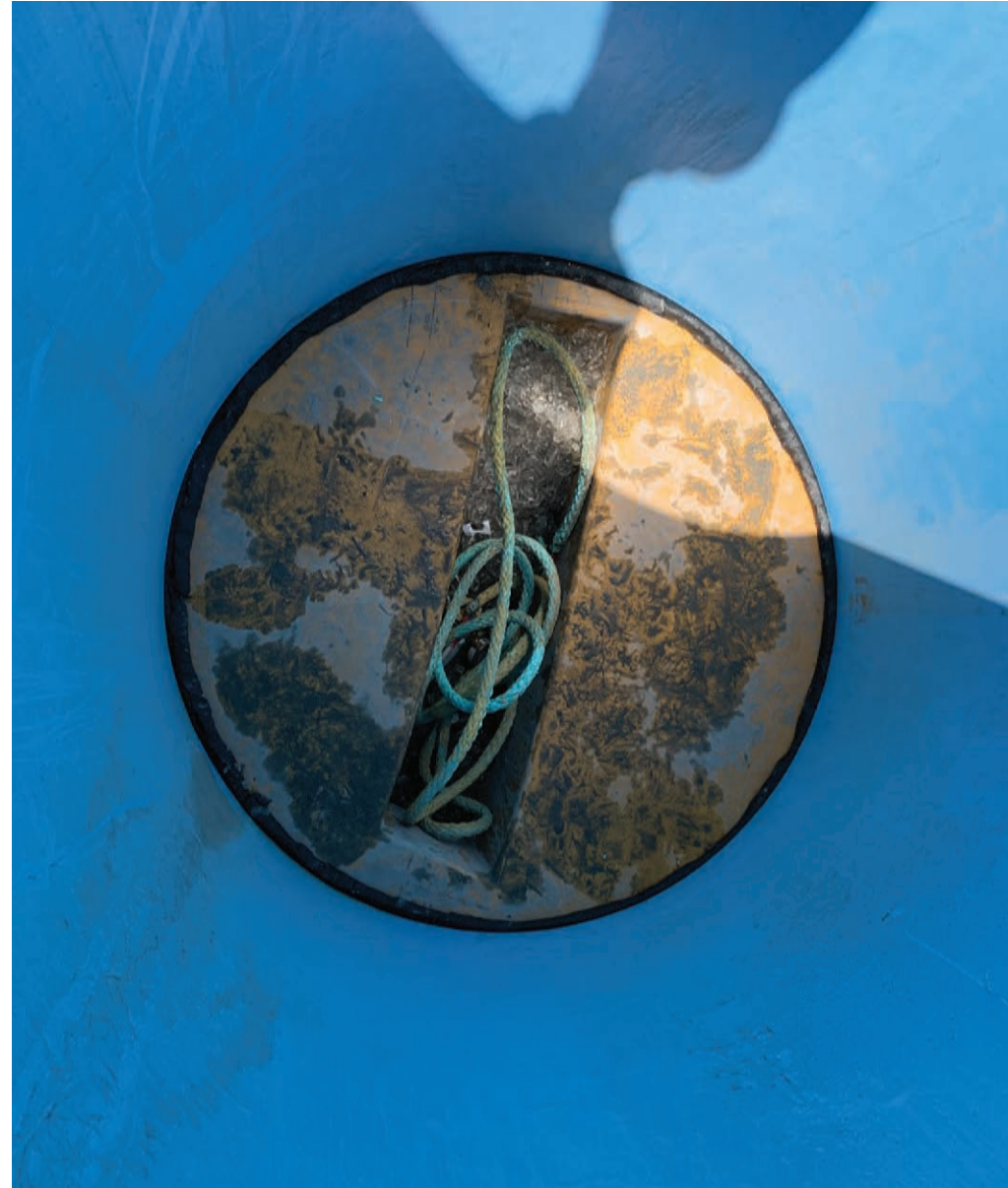
ENSURE RISER IS SEALED ON FRP BASELINER JOINT, ENSURING MASTIC SEALANT IS FULLY ENGAGED
