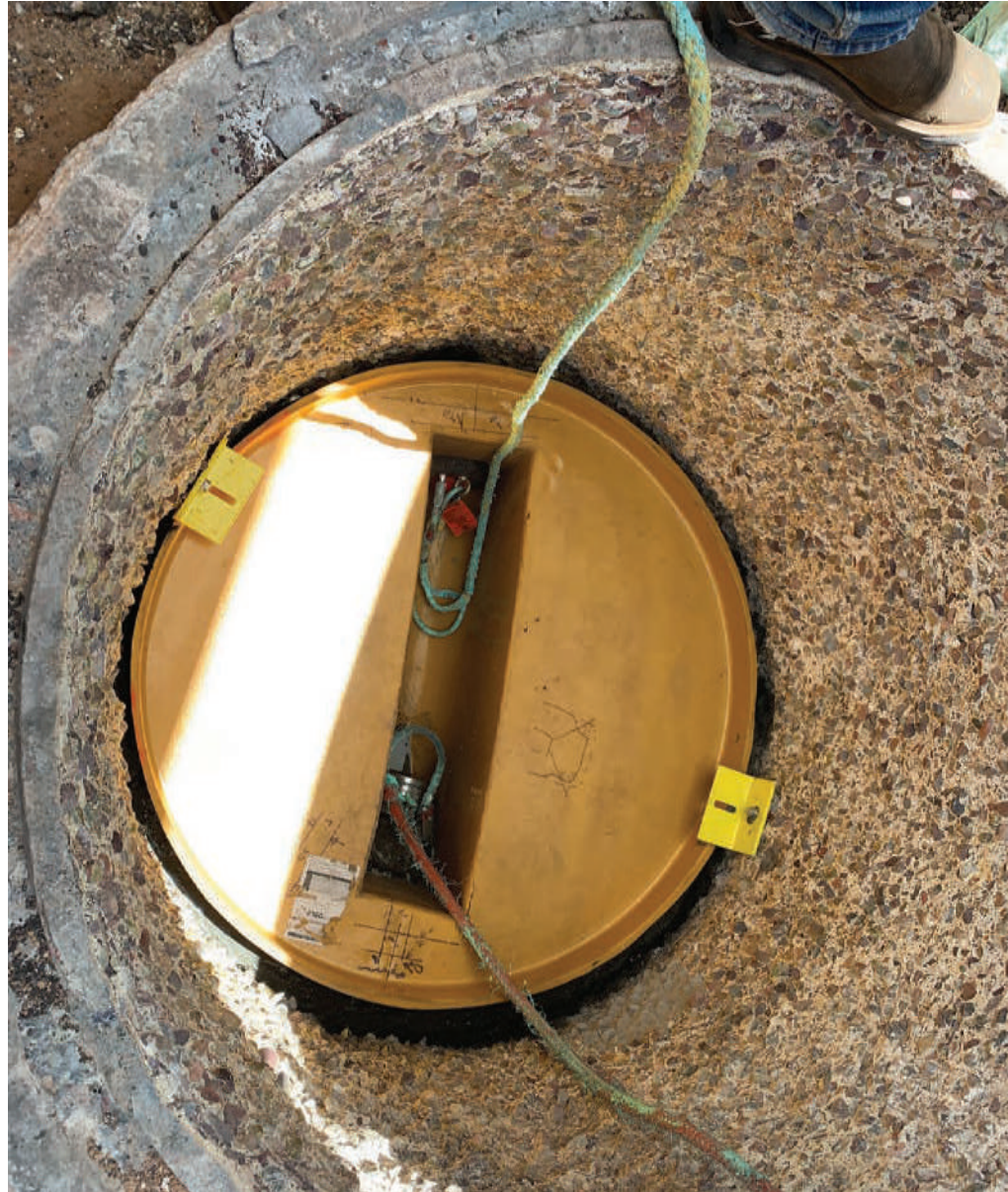
SECURE LINER IN PLACE
