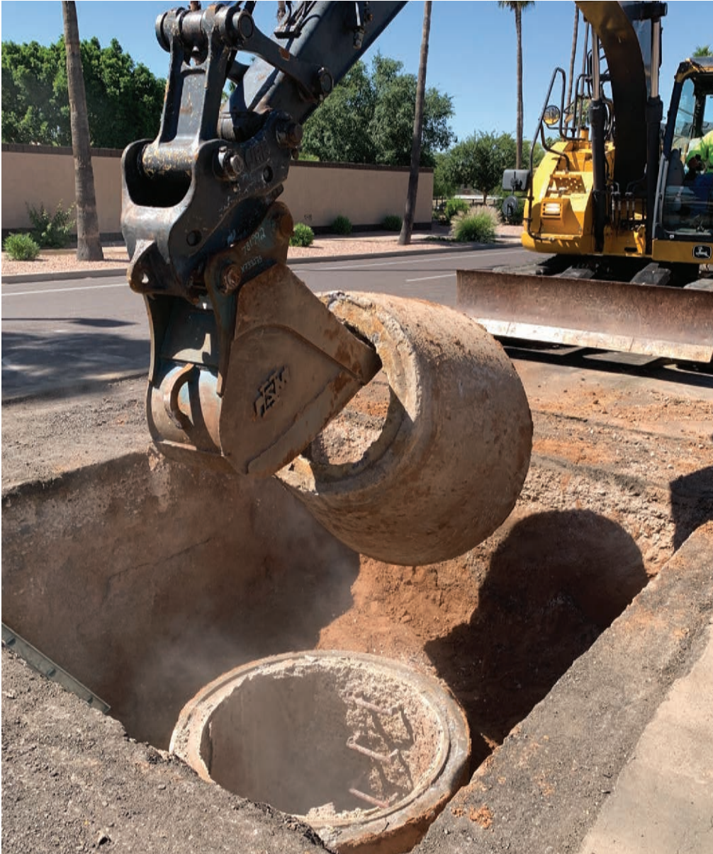
EXCAVATE AND REMOVE EXISTING FLAT TOP OR CONE TOP
