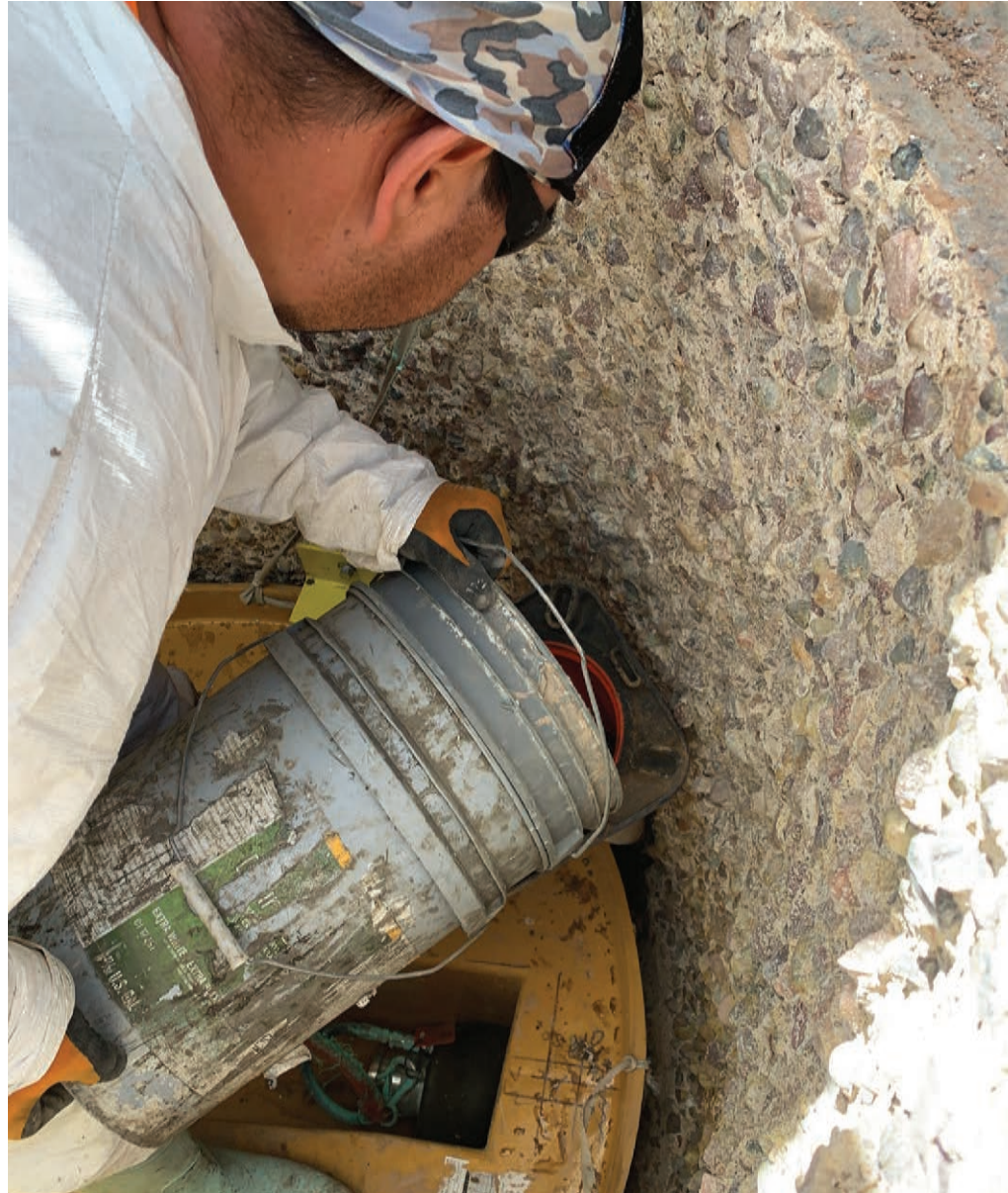
POUR HIGH FLOW, NON SHRINK GROUT BEHIND LINER
