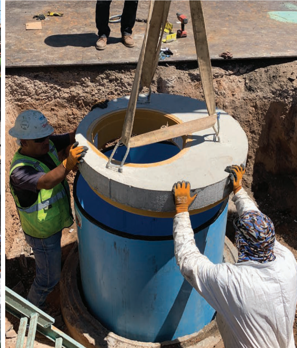
LOWER FRP LINED PRECAST LID ONTO RISER
