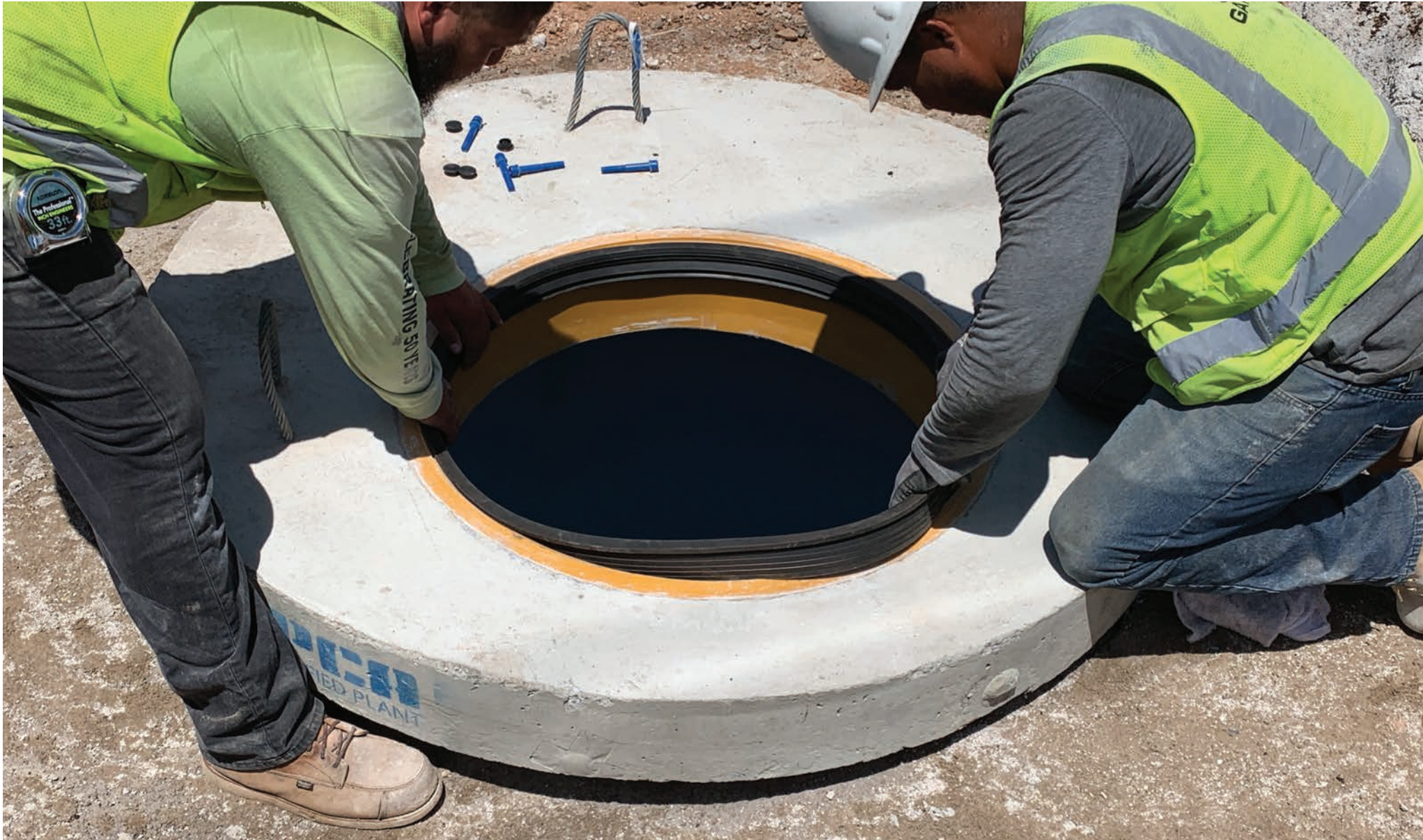
INSERT TELESCOPIC ACCESS COLLAR (TAC) GASKET
