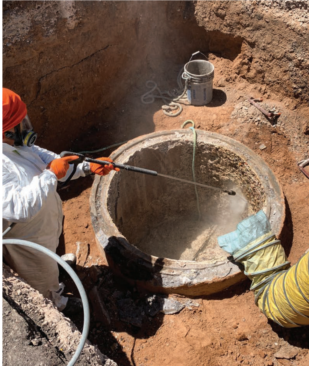
CLEAN ALL MH WALLS. SUBSTANTIALLY REMOVE INCONTINENT CONCRETE MATERIAL
