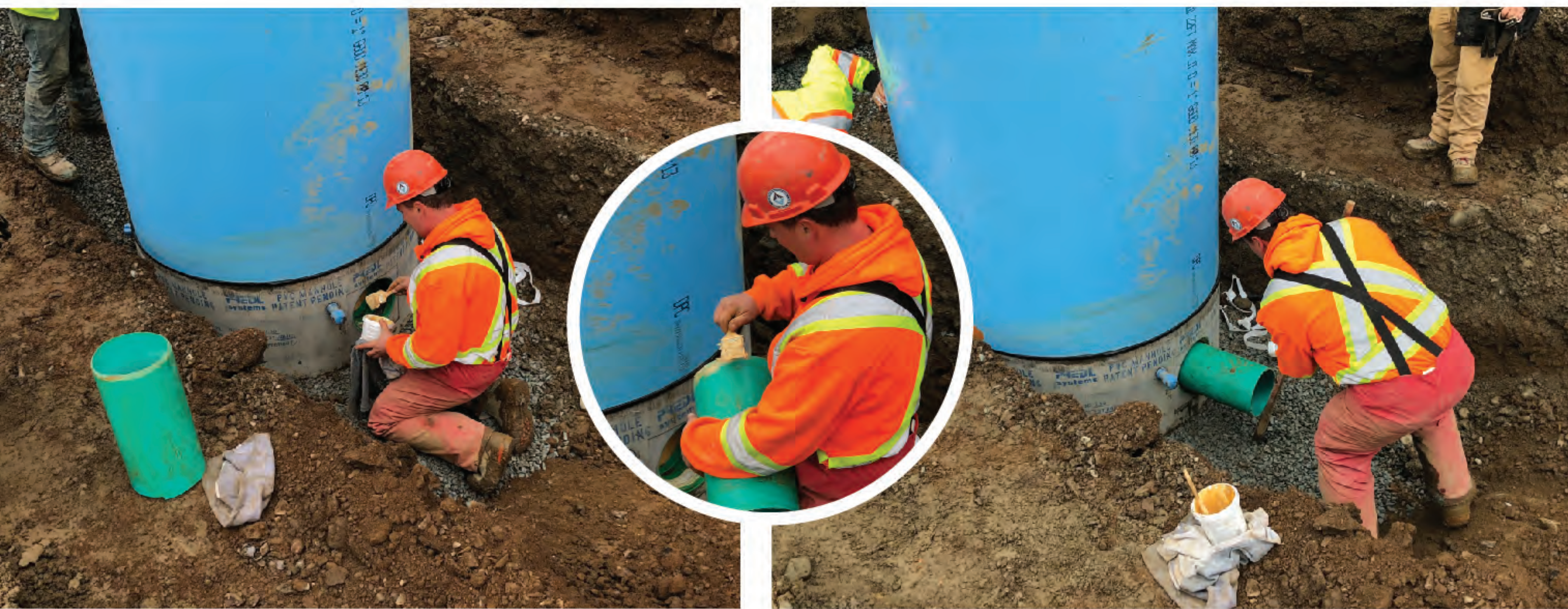
STUB-OUT OF INLET
