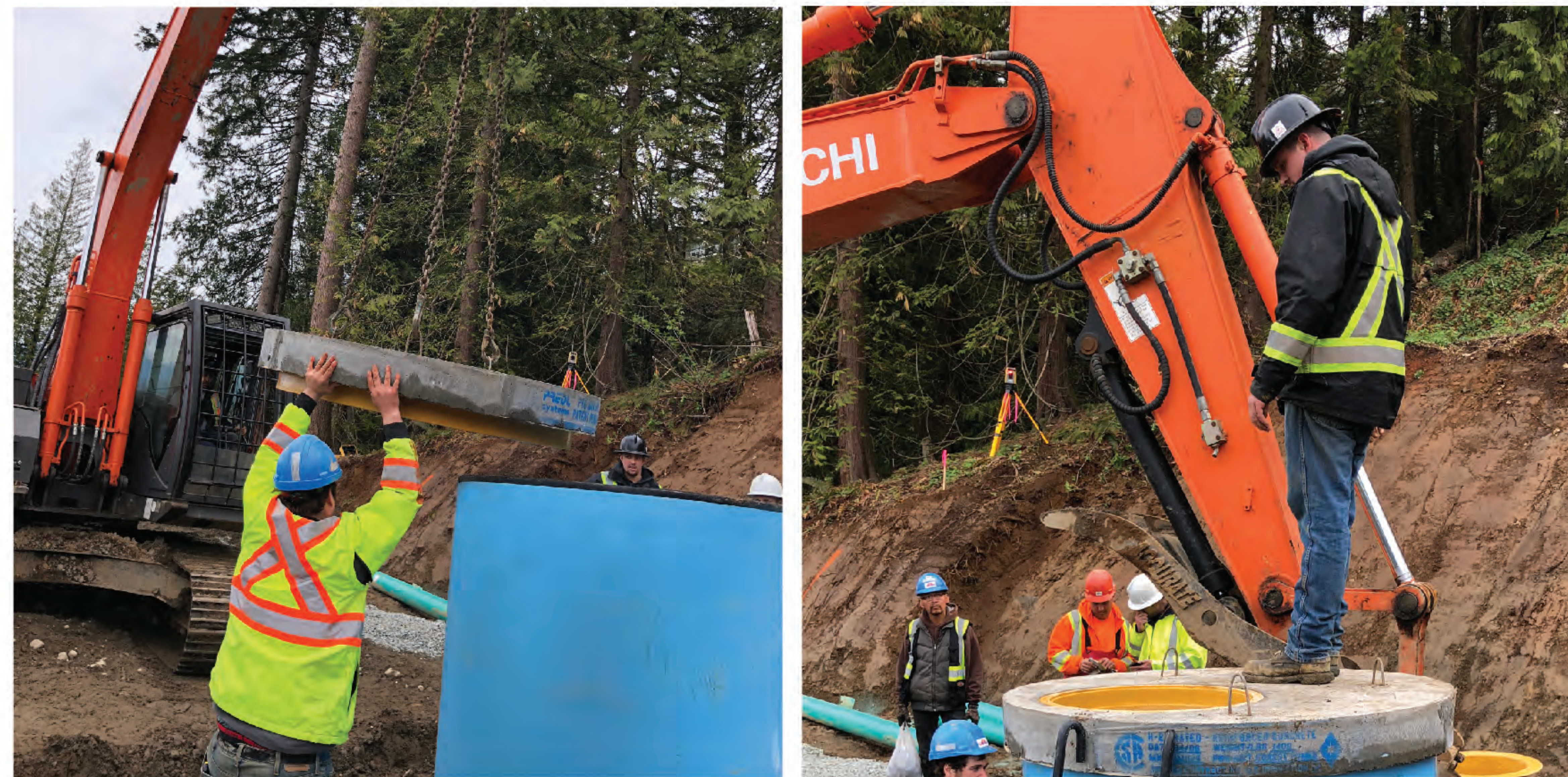
INSTALL H-20 RATED ASTM C478 PRECAST MH LID w/ INTEGRAL PREDL FRP LINER & TELESCOPIC ACCESS COLLAR (NOT SHOWN)
