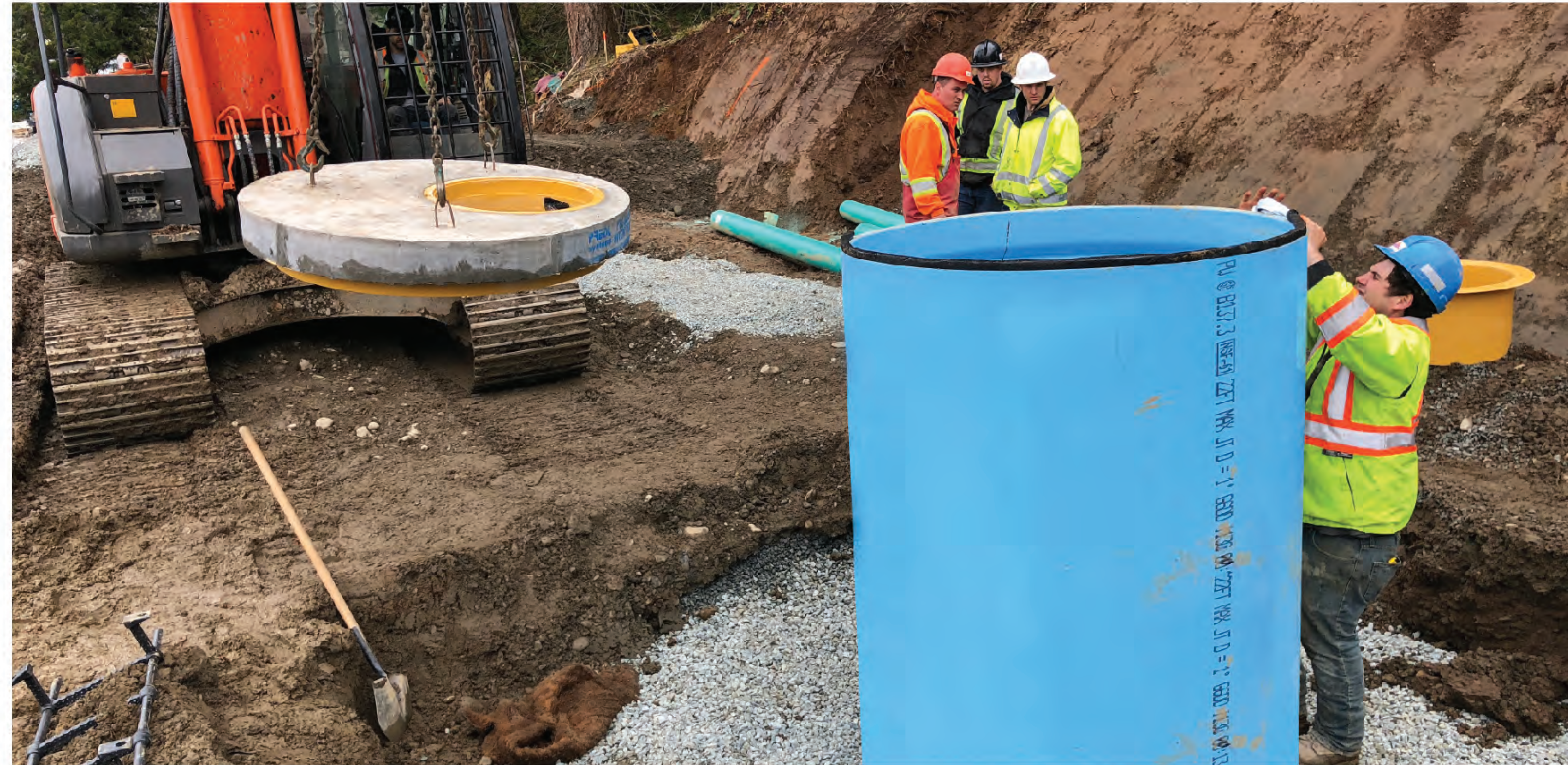
ASTM C990 BUTYL RUBBER MH JOINT SEALANT
