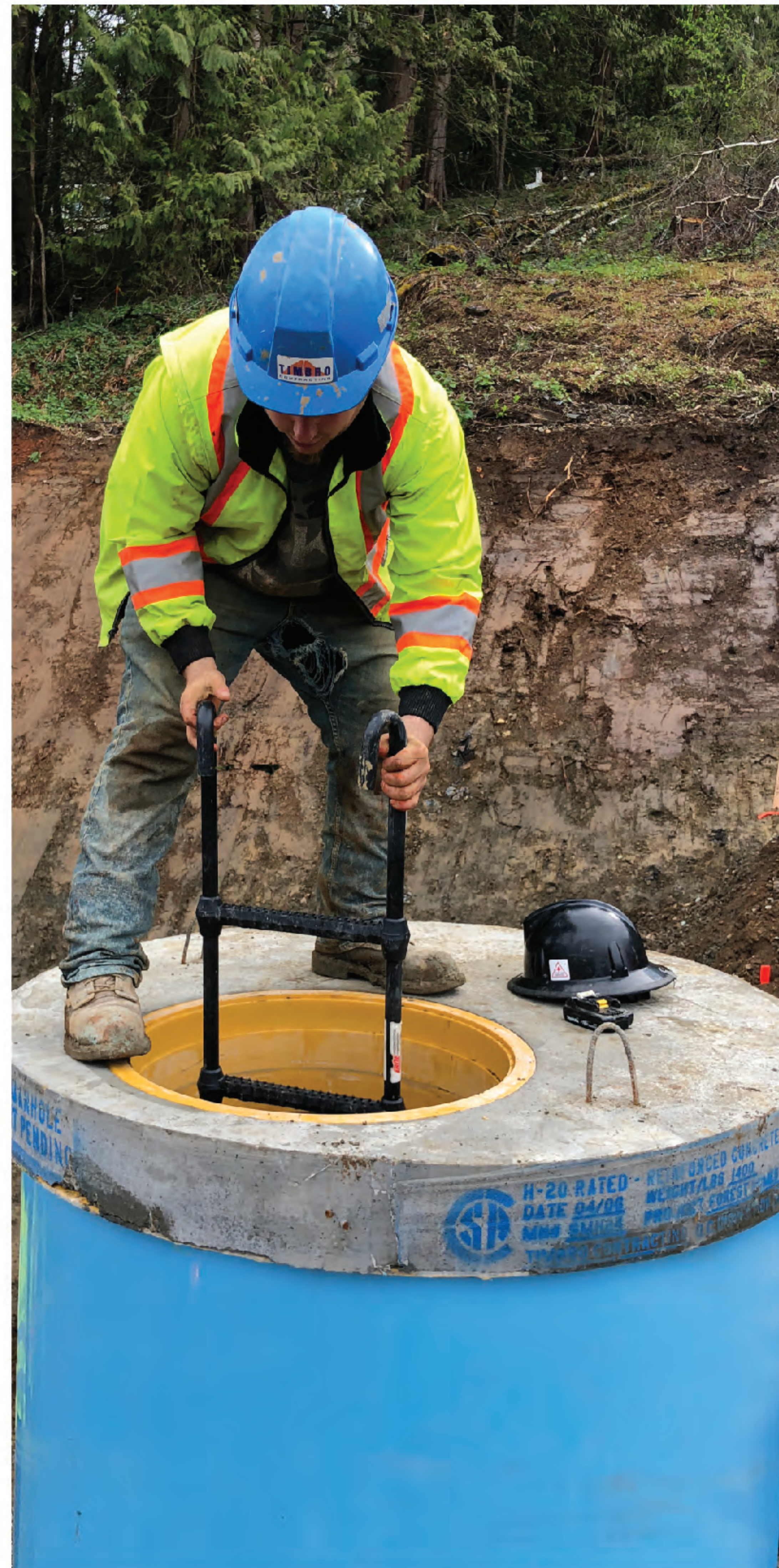
MH LADDER INSTALLATION - REQUIRES SS316 HARDWARE w/ O-RINGS
