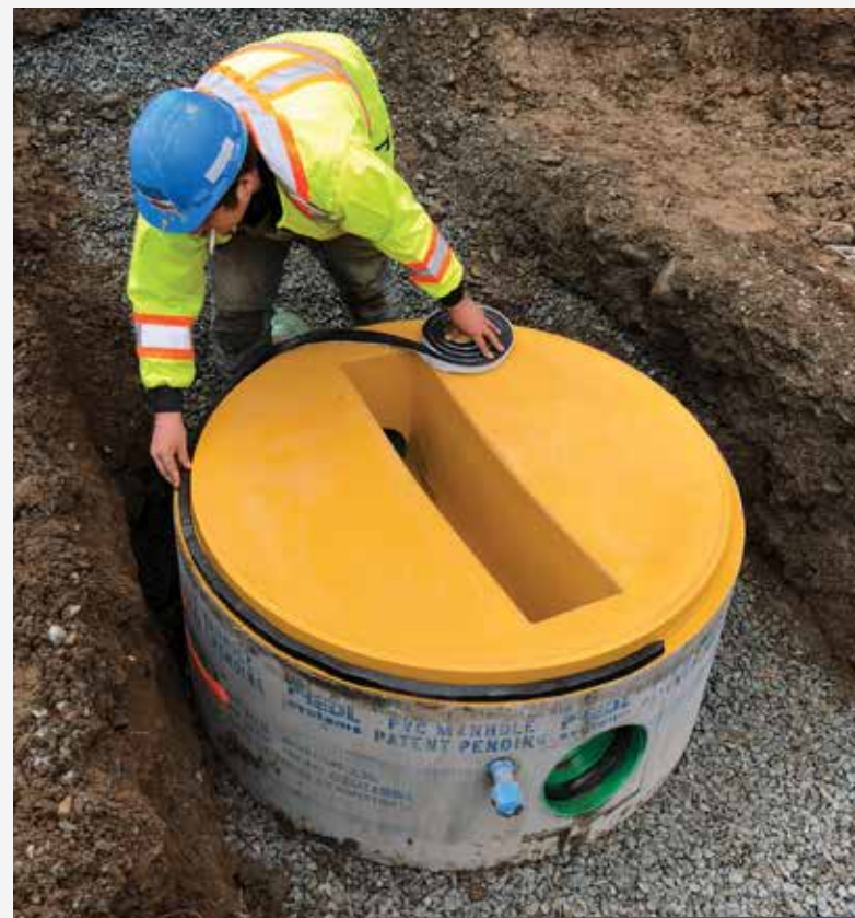
ASTM C990 BUTYL RUBBER MH JOINT SEALANT
