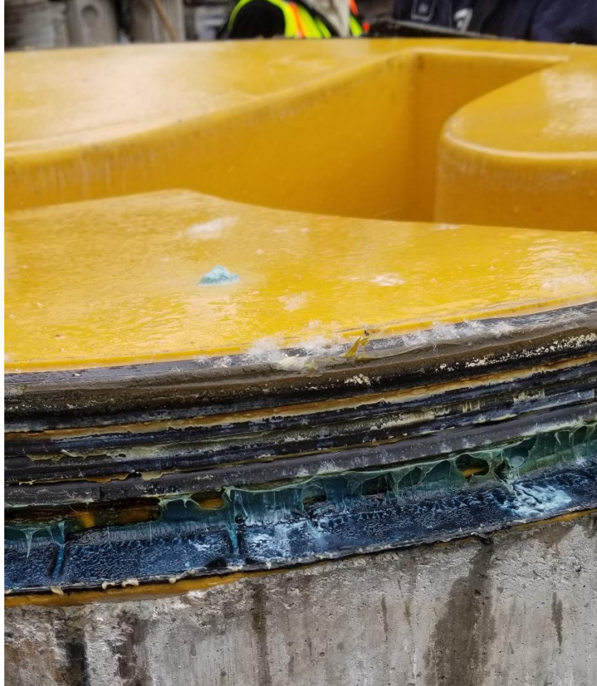
Pic.10: Gasket on vertical interface of concrete and PVC pipe and Mastic on Horizontal surface of concrete
