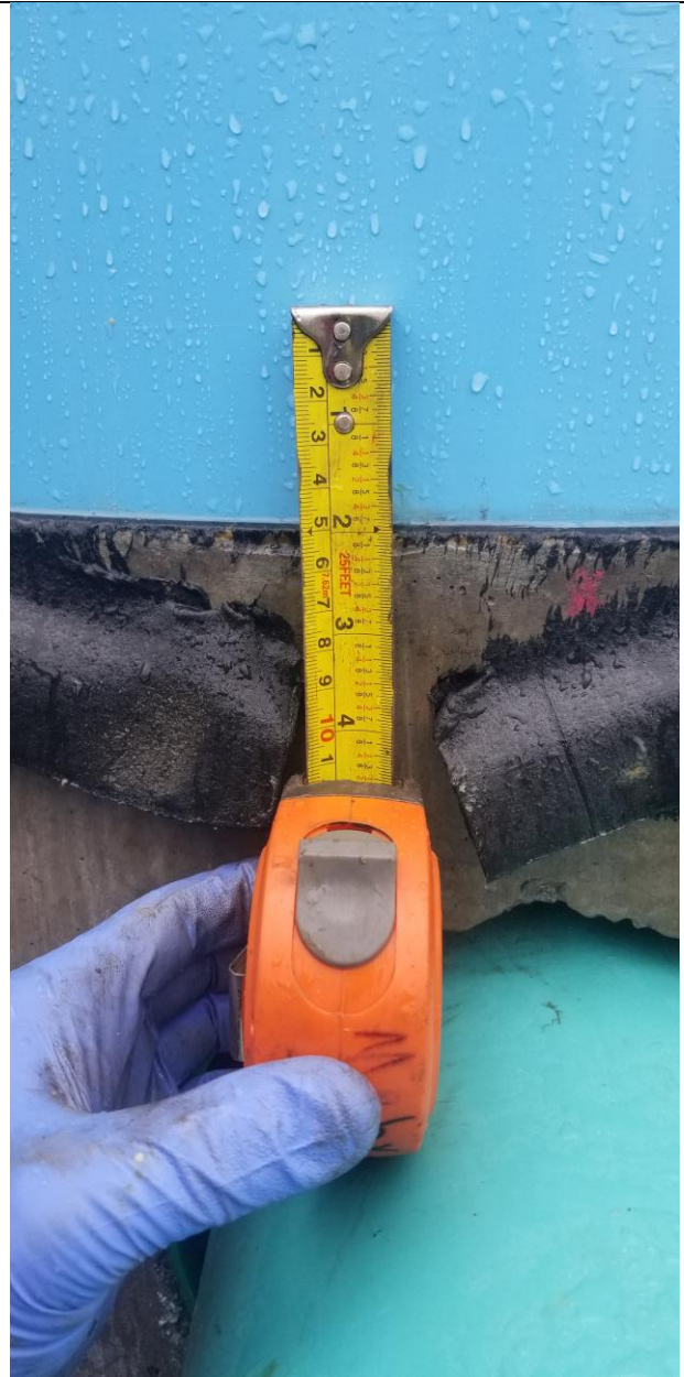
Figure 5- Installed mastic (Assembly configuration 2). 1-2 mm thickness after installing the concrete cap
