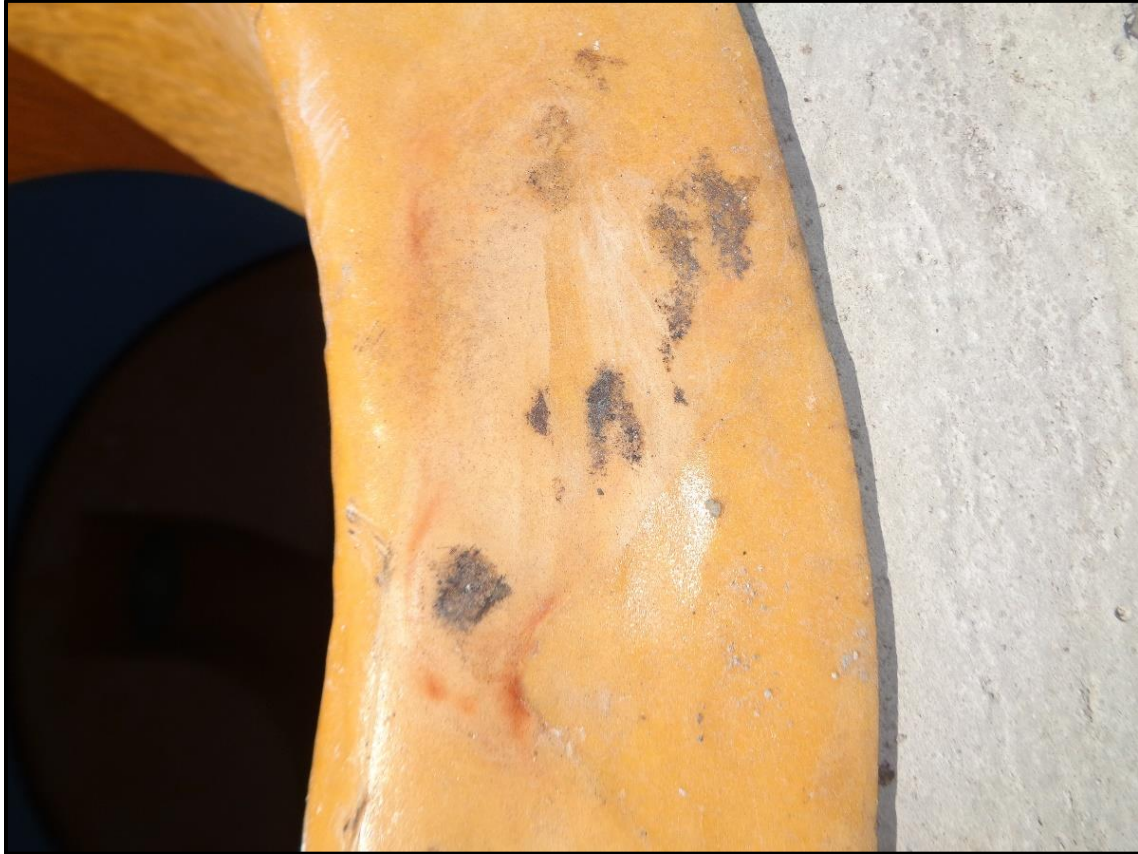
Pic.7 Local contact marks on the fiber glass collar under the concrete rings, does not indicate any signs of the failure the concrete rings
