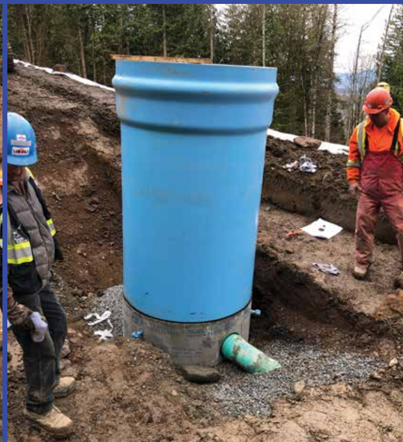
1200mm (48") ID DIAMOND PLASTICS DR51 PVC PIPE RISER SET TO MH BASE
