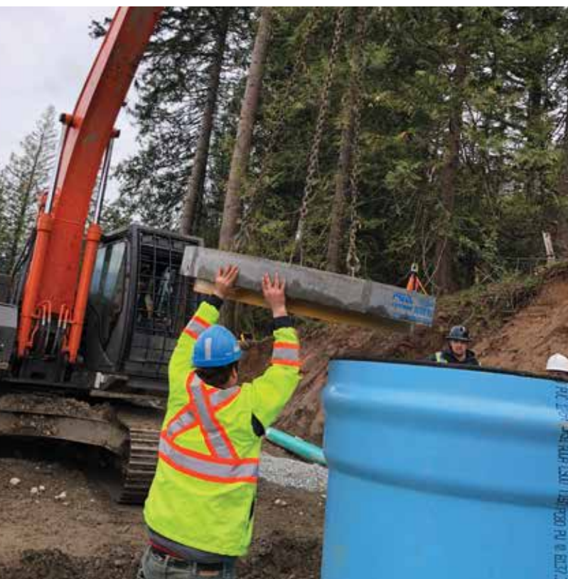
INSTALL H-20 RATED ASTM C478 PRECAST MH LID w/ INTEGRAL PREDL FRP LINER & TELESCOPIC ACCESS COLLAR (NOT SHOWN)
