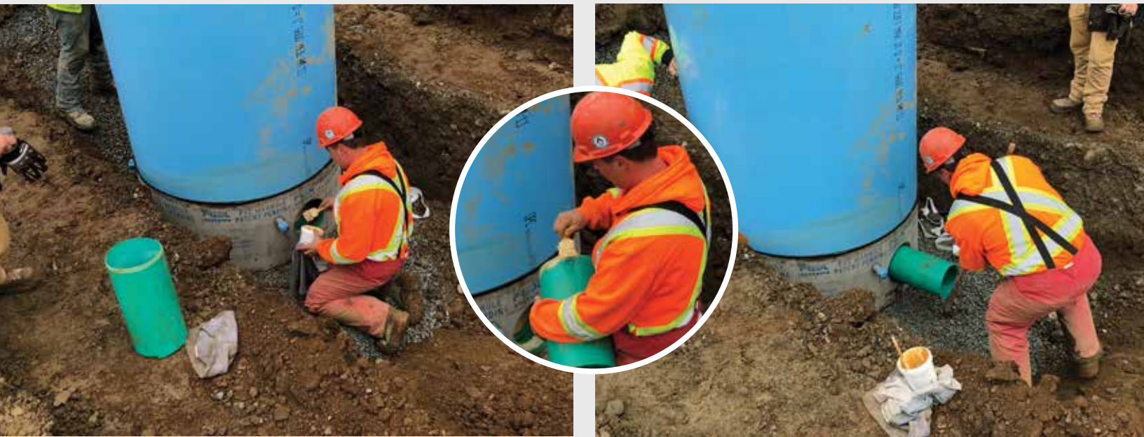
STUB-OUT OF INLET
