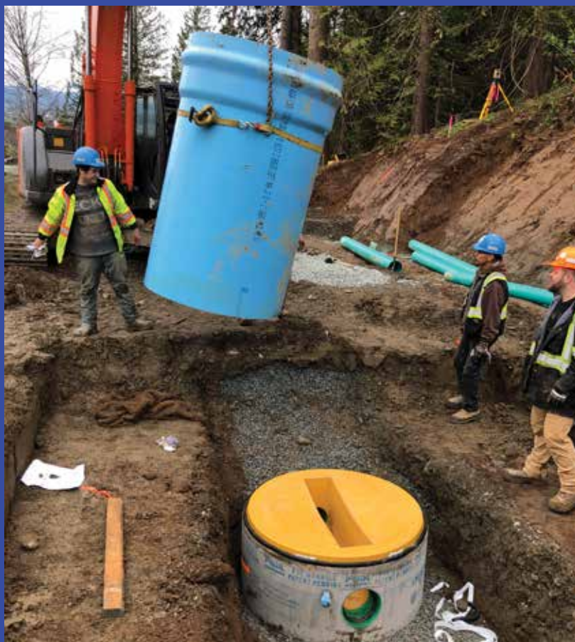
1200mm (48") ID DIAMOND PLASTICS DR51 PVC PIPE RISER SET TO MH BASE
