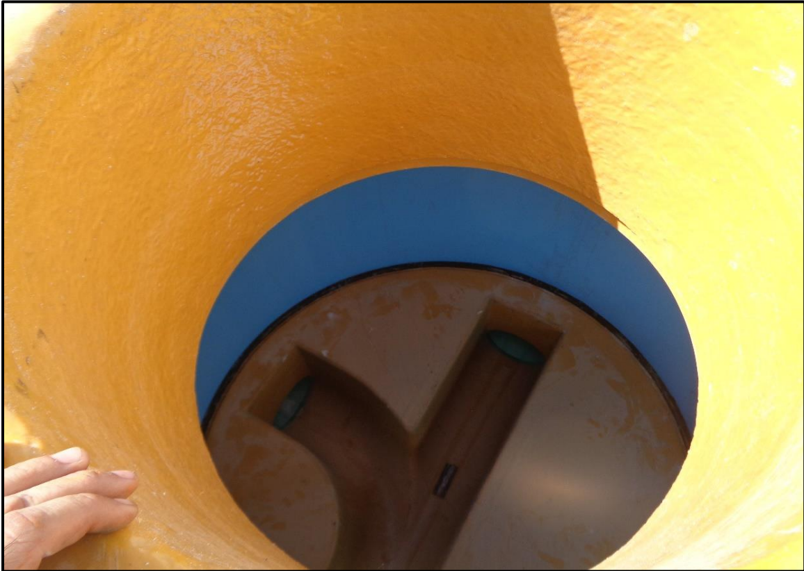
Pic.8: Inside view of manhole after testing
