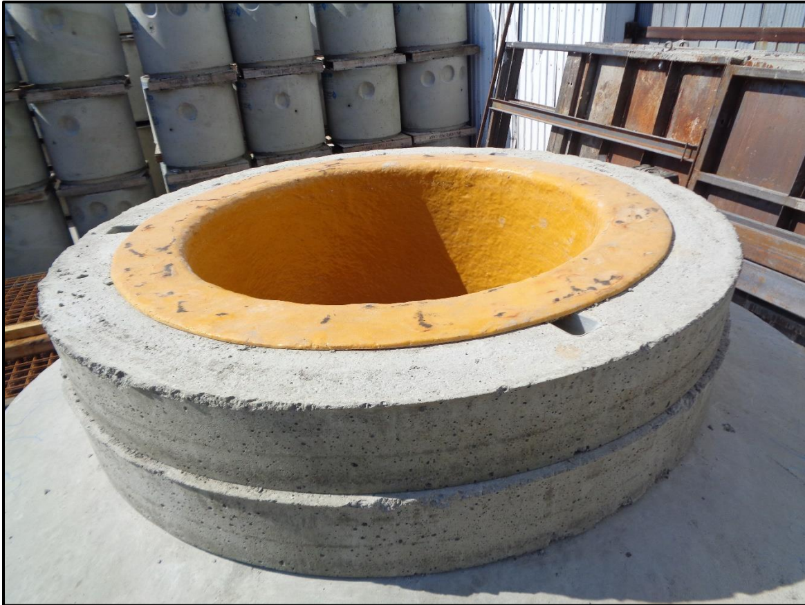
Pic.6: Local contact marks on the fiber glass collar under the concrete rings, does not indicate any signs of the failure
