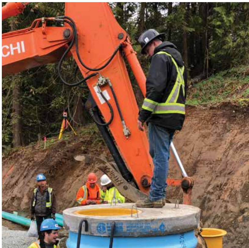
INSTALL H-20 RATED ASTM C478 PRECAST MH LID w/ INTEGRAL PREDL FRP LINER & TELESCOPIC ACCESS COLLAR (NOT SHOWN)
