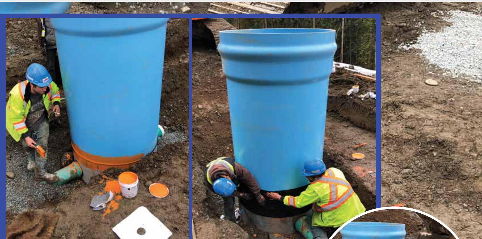
ASTM C877-COMPLIANT EXTERNAL MH JOINT WRAP (INCLUDES PRIMER)
