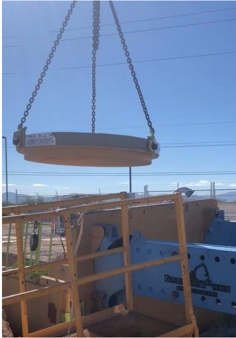
Figure 5 Manhole adjusting ring Installation
