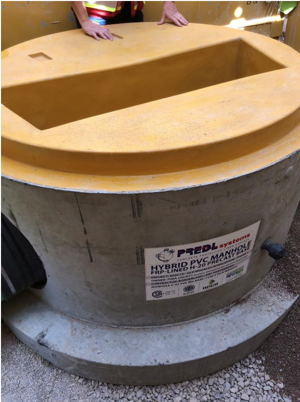
Figure 4 Manhole base (note added weigh ring to prevent buoyancy)
