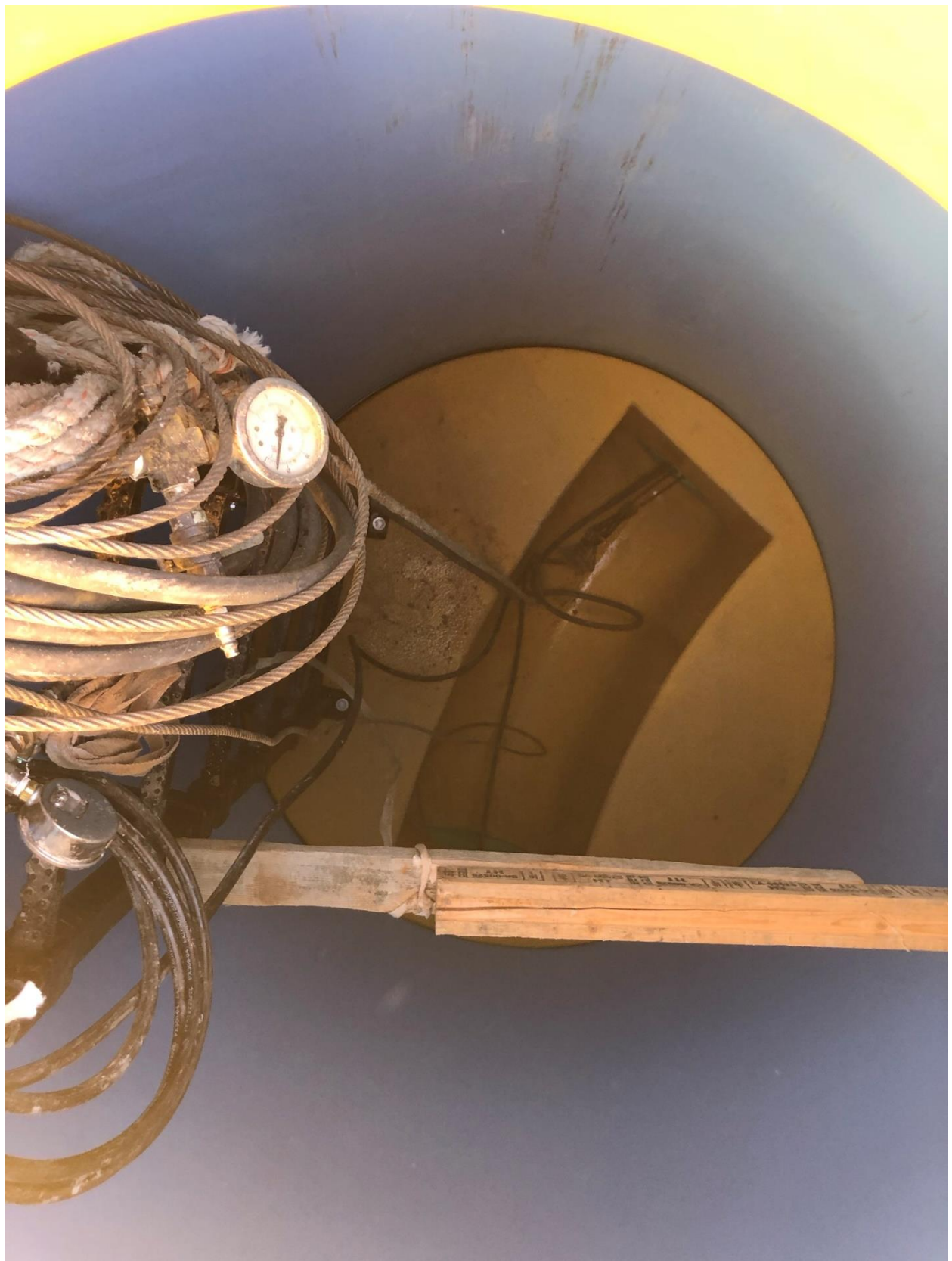
Figure 10 Manhole pressure testing photos
