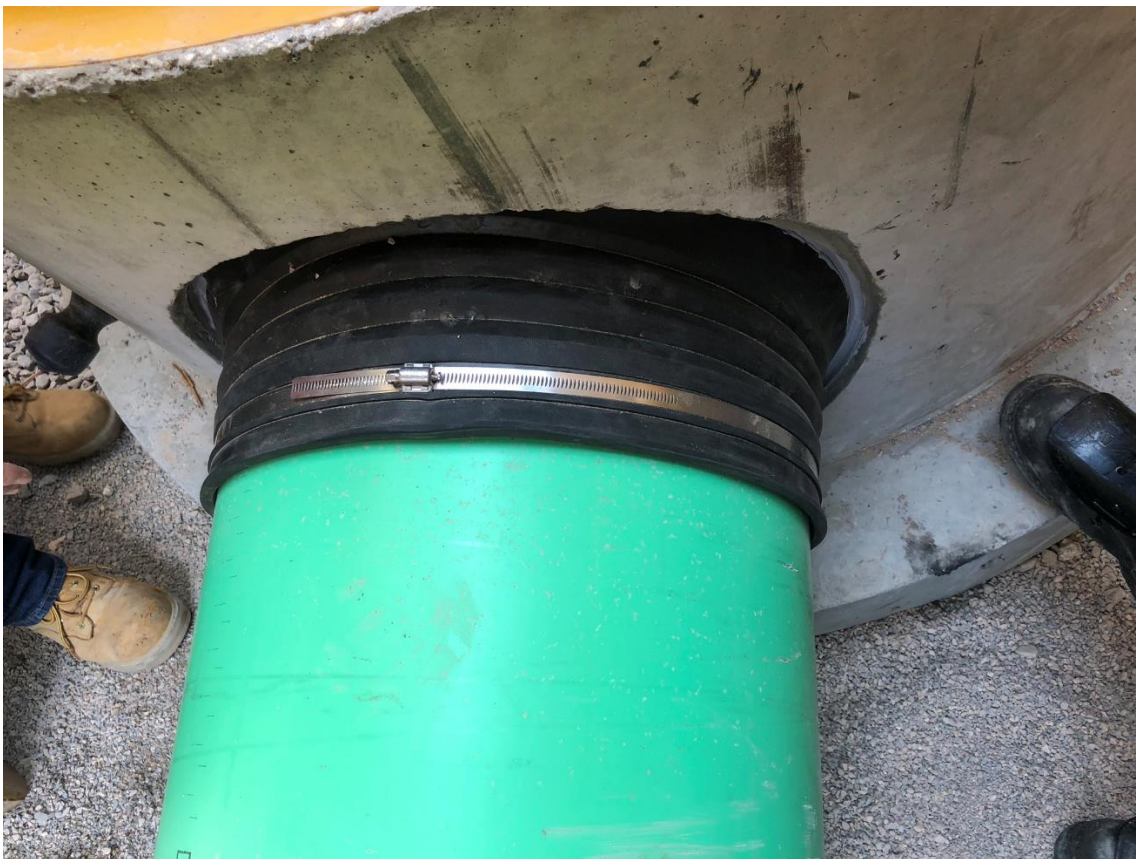
Figure 2 Pipe boot strap
