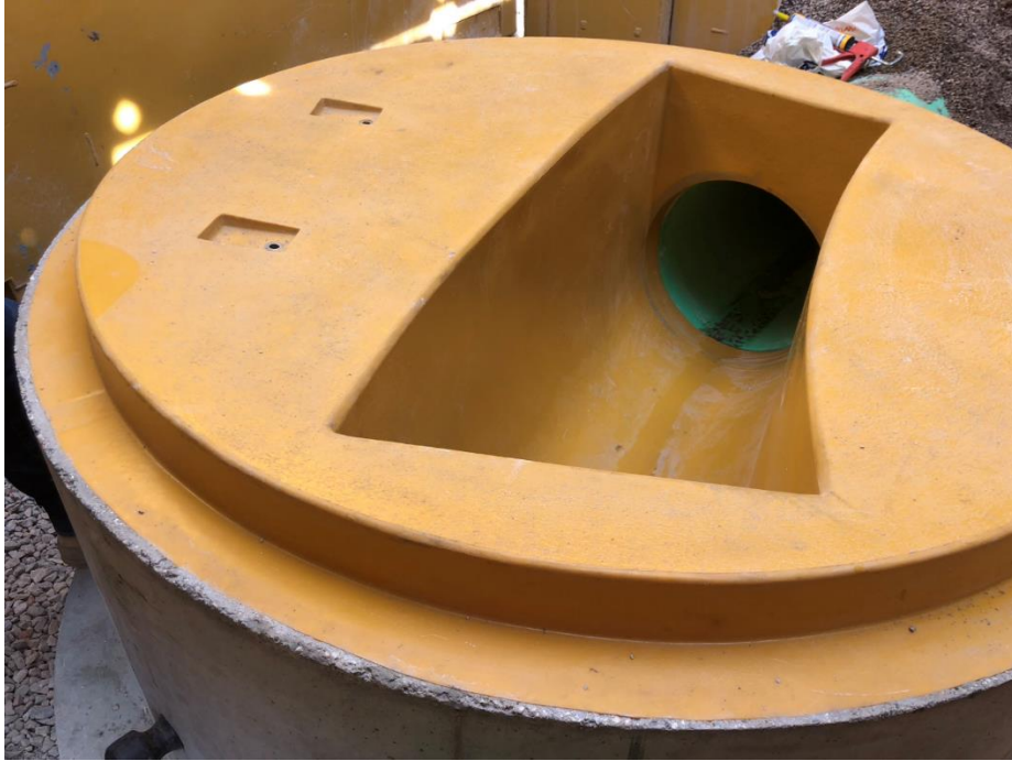
Figure 1 Manhole base with FRP liner
