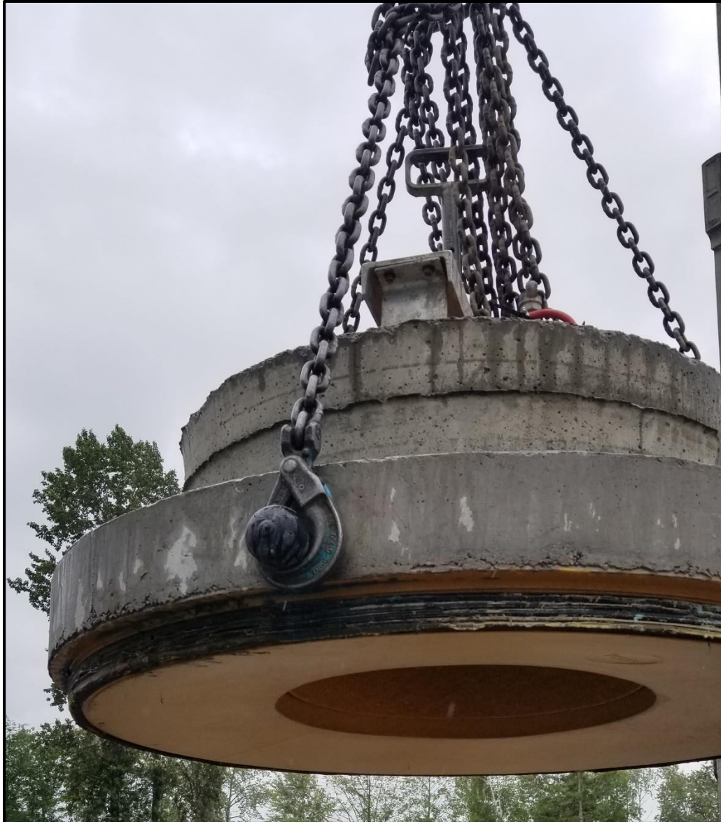
Pic.9: Gasket on vertical interface of concrete and PVC pipe
