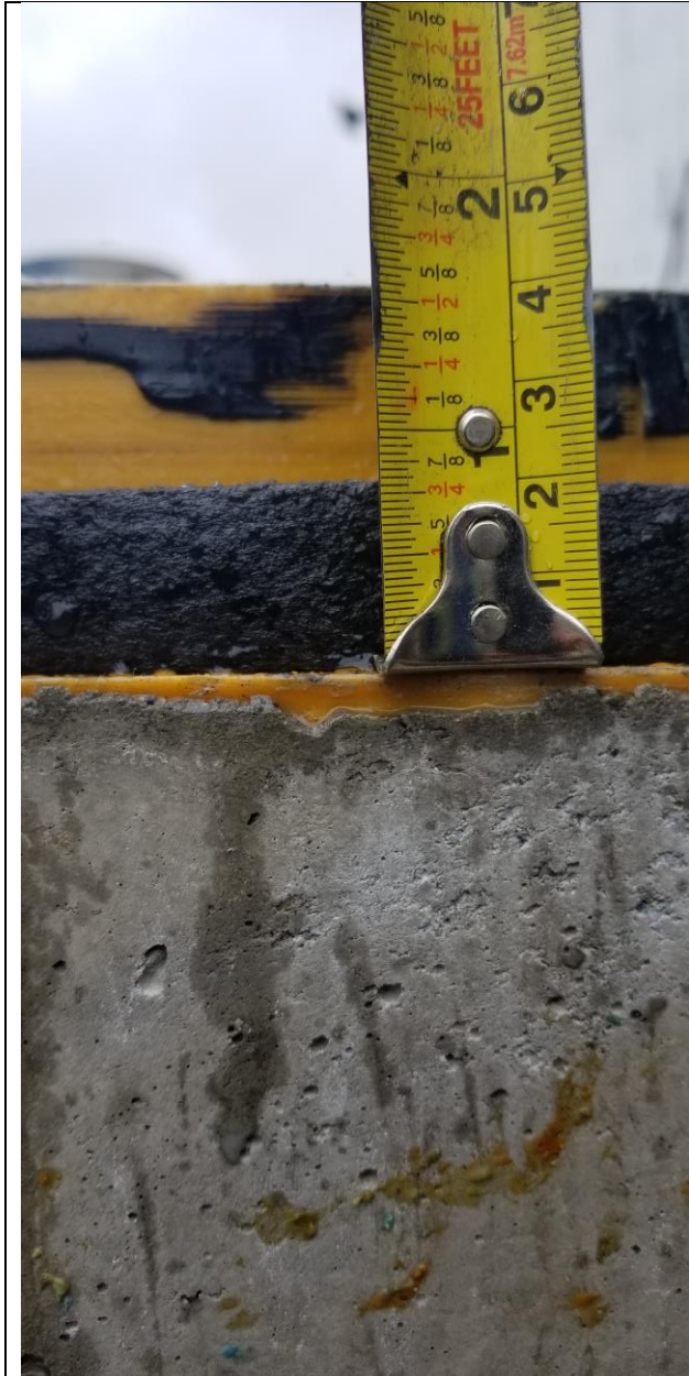
Figure 4- Installed mastic (Assembly configuration 2). 19 mm thickness before installing the concrete cap
