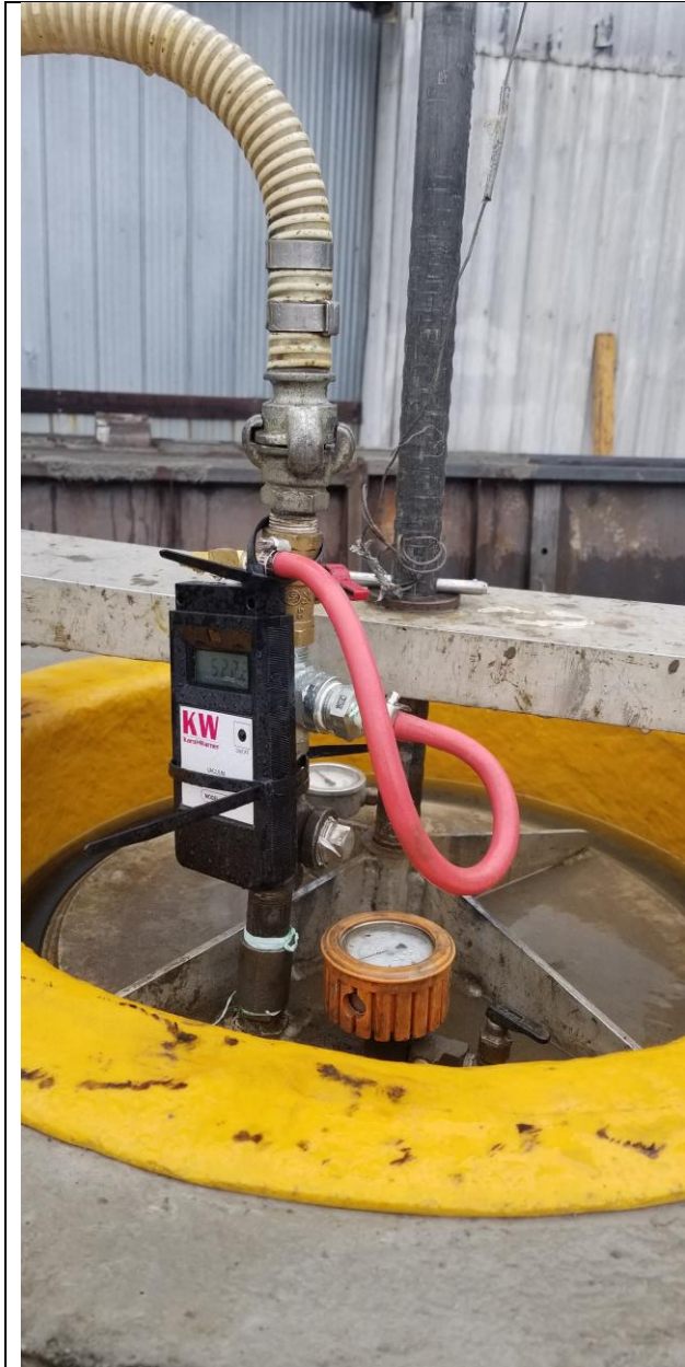
Figure 2- Installed lid with vacuum rubber
